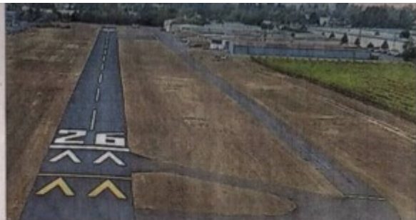
The skypark's newly paved runway.
